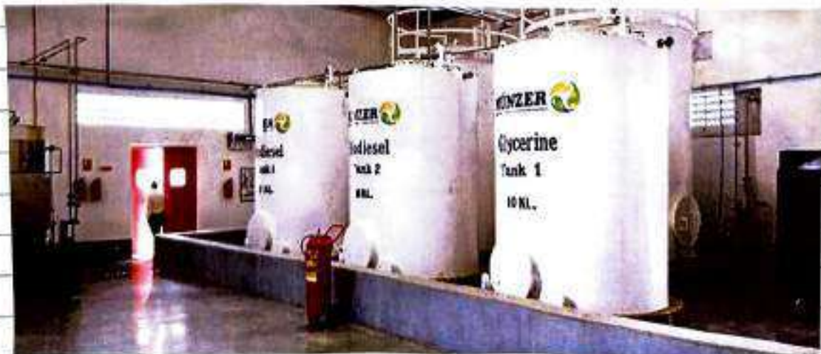
After processing Glycerin & Biodiesel transferred FOR EDUCATIONAL USE to the tanks.
